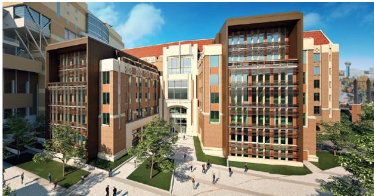
Construction has begun on the new $129M Engineering Complex to house NE and their 23 new laboratories. See progress: tiny.utk.edu/gateway
